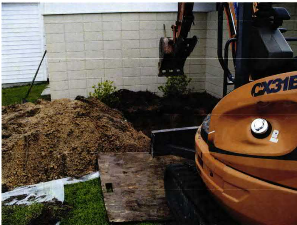
Picture 2: UST 1255Dove removal in progress.
